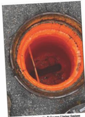
Figure 1. OBIC Composite Polyurea Lining System
